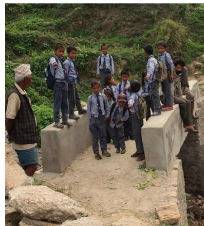
A bridge at Lulu VDC, Kalikot
