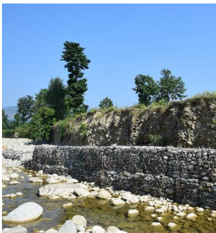
Gabion wall at Sugarkhal VDC, Kailali
