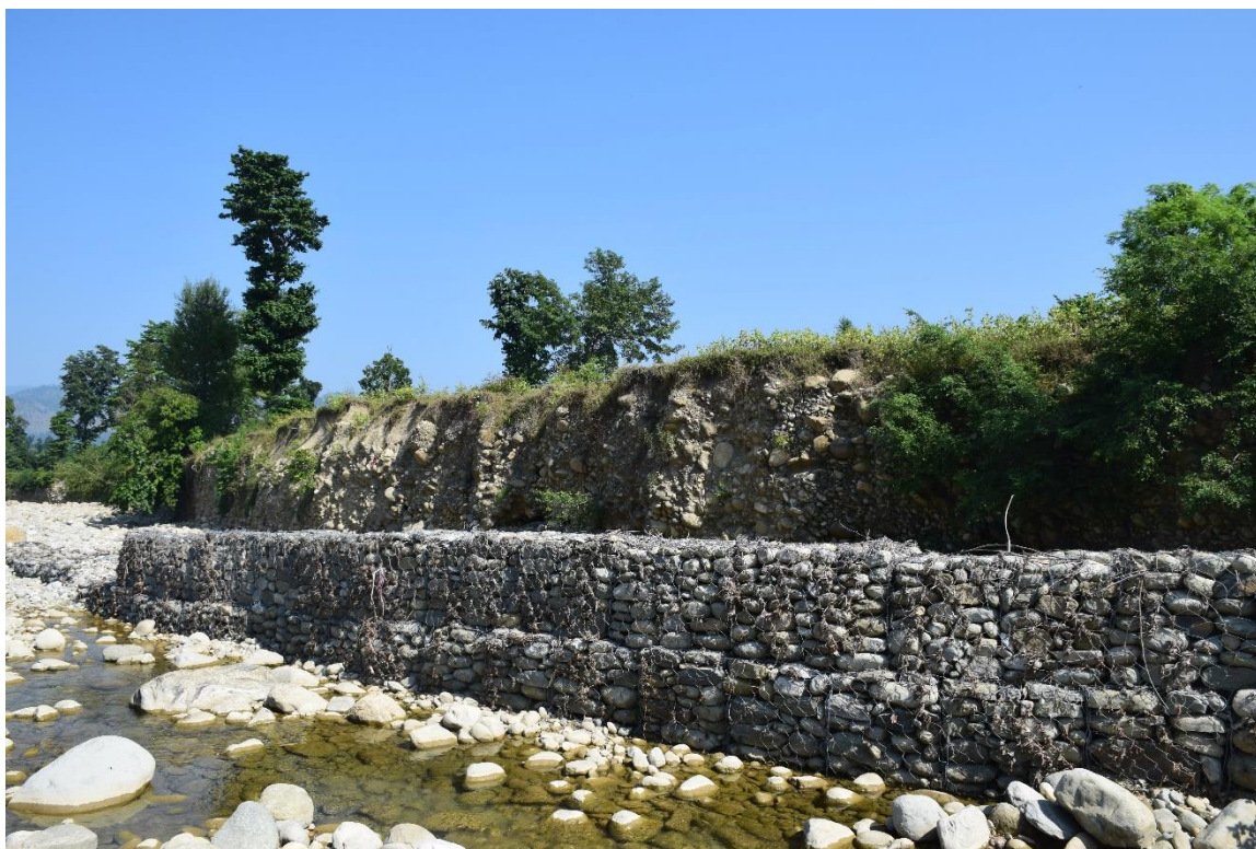
Gabion wall constructed in Sugarkhal VDC, Ward no.9, Kailali
